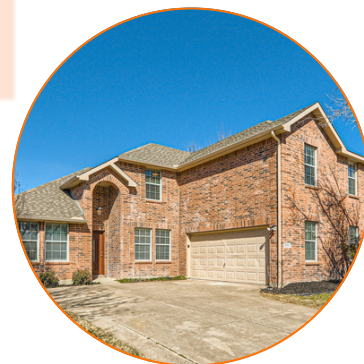
902 Marble Creek: A BIG Investor renovation with foundation repair!
