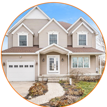
13312 N Clio Road: Incredible transformation of an unmaintained home!
